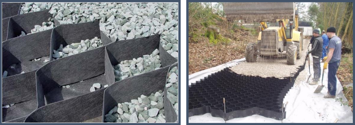
Figure 9 Examples of Cellweb filling with angular stone
